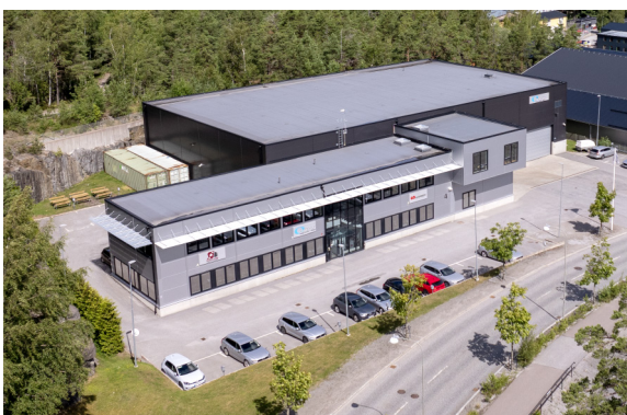
Head office and warehouse
