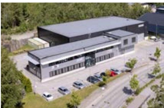
Head office and warehouse
