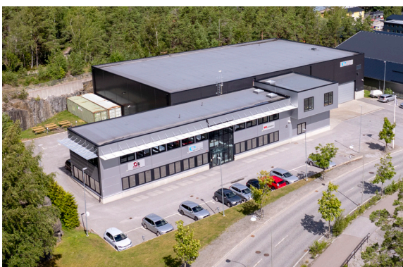
Head office and warehouse
