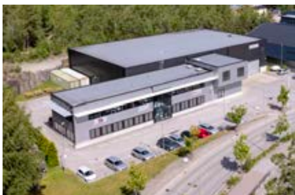
Head office and warehouse
