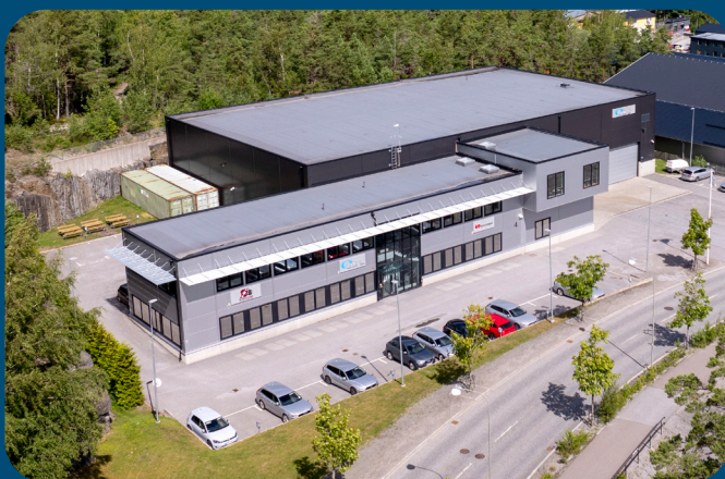
Head office and warehouse
