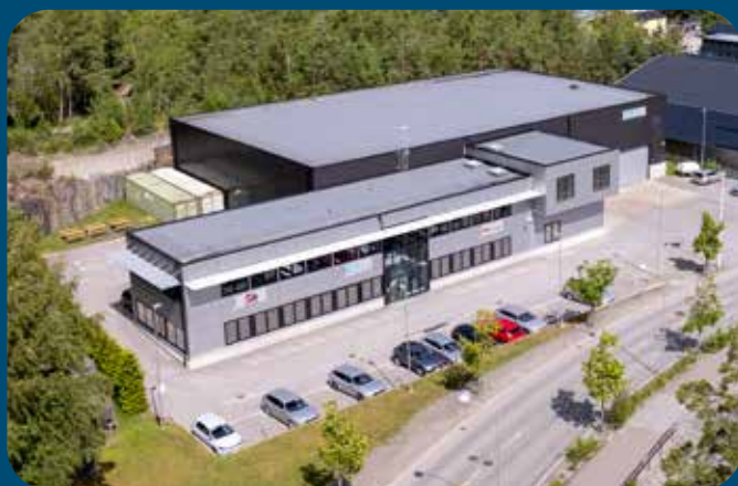
Head office and warehouse
