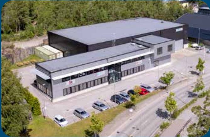
Head office and warehouse
